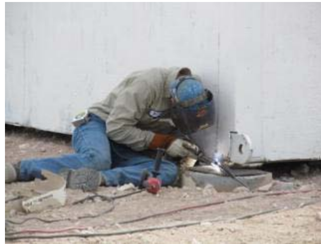
Typical HRM off-loading, final positioning, and securing to support pilings
